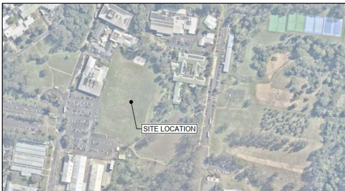
Plate 2: Air View of the Project / Site Location at SCU
