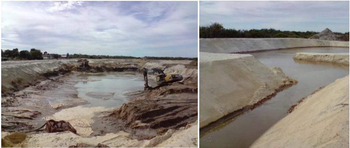
Figure 4.7 Open excavation of canal infrastructure with dewatering sump pump in foreground and recharge trench with settling basin.
