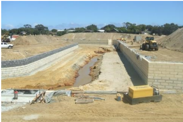
Figure 4.9 Wall construction underway within central canal.
