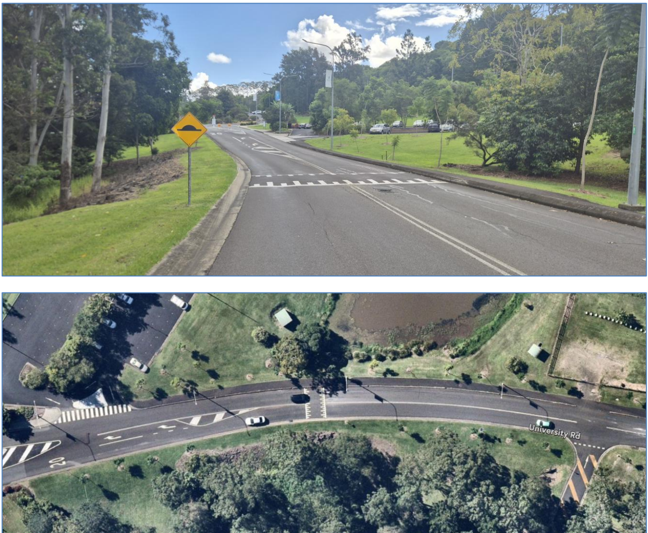
Figure 2.2: University Road (view westbound)
